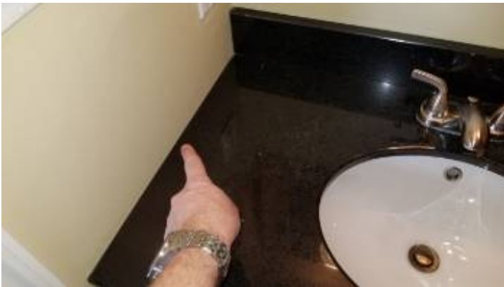
Missing/insufficient caulk.
