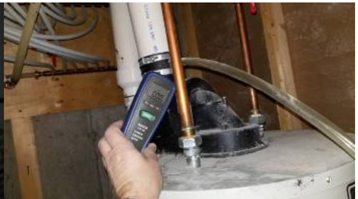
Carbon monoxide reading of 0.
