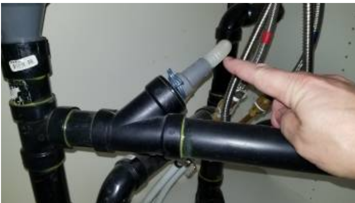
No high drain loop.
