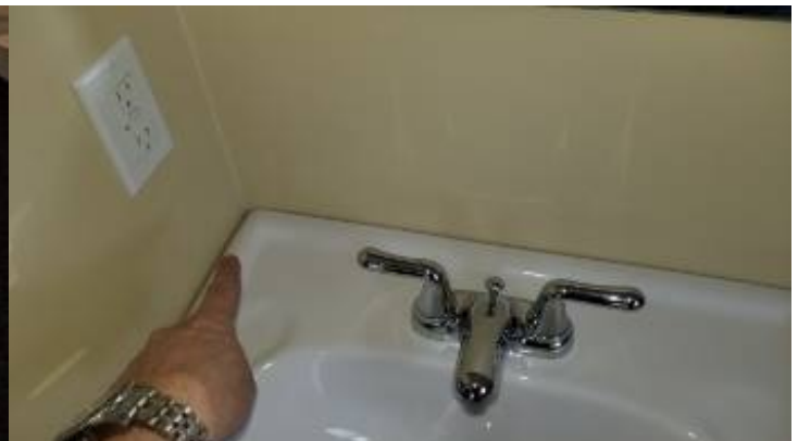
Missing/insufficient caulk.
