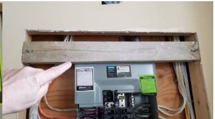
Inaccessible screws.
