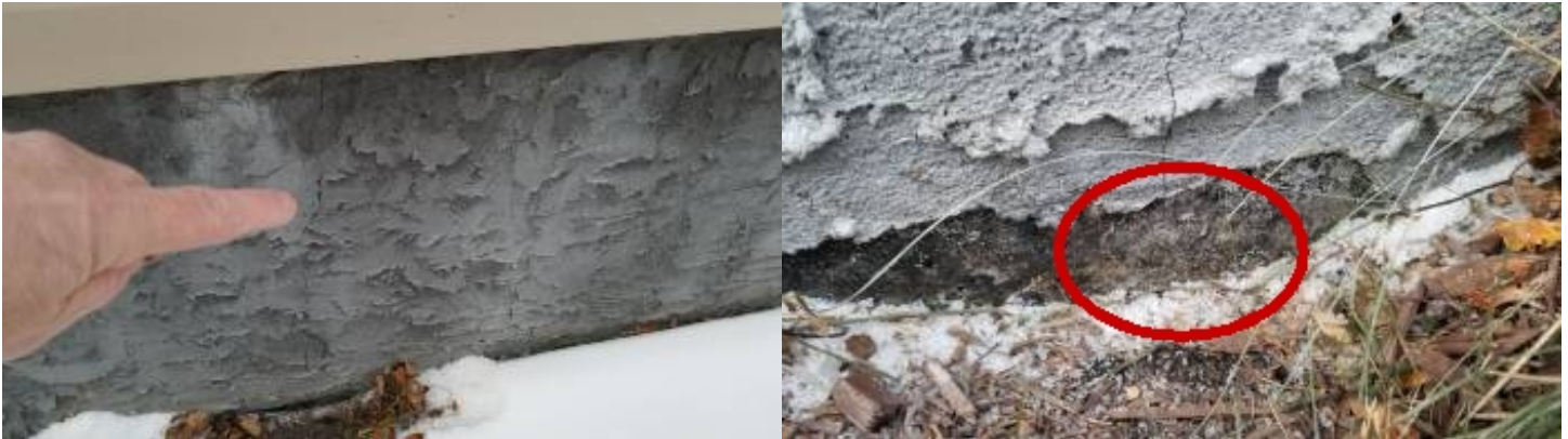
Cracked parging.
