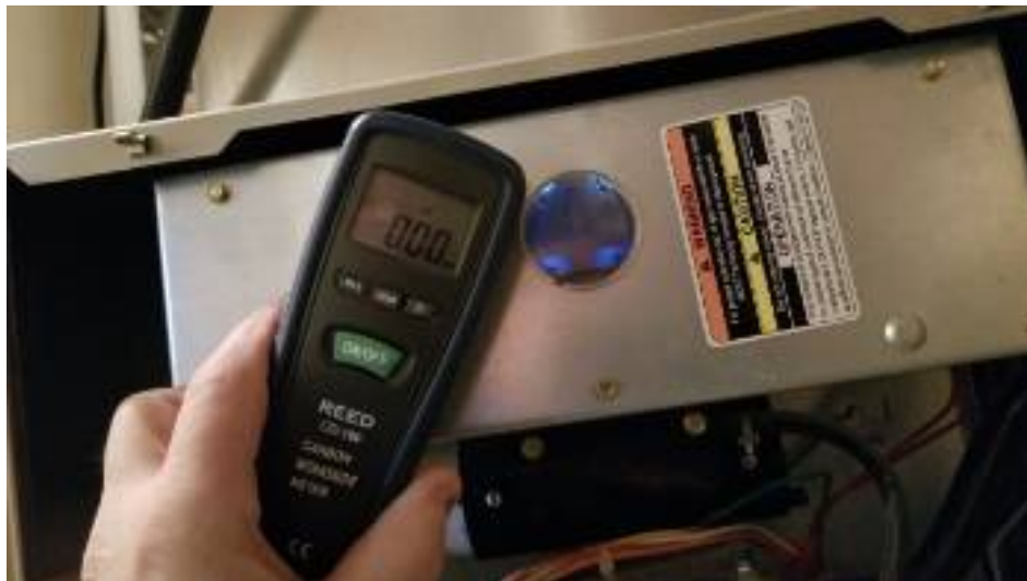
Carbon monoxide reading of 0.
